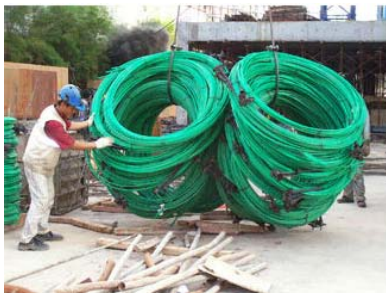
Gambar-7: Gulungan strand Gambar-8 : Marking posisi strand
