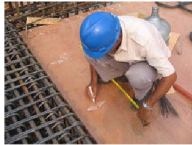
Gambar-7: Gulungan strand Gambar-8 : Marking posisi strand
